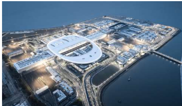
Hong Kong-Zhuhai-Macao Bridge
